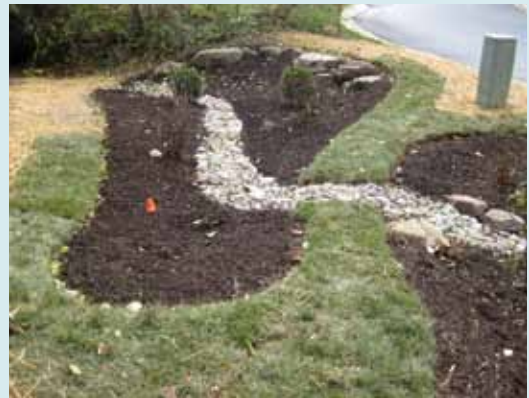
2-celled rain garden just after installation
